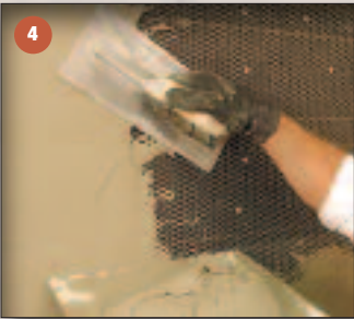
Apply mortar for scratch coat.
