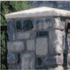
29" L x 29" W x 2.25" Thick 4.75" Thick at Center Point
