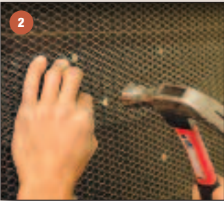
Install corrosion resistant metal lath.
